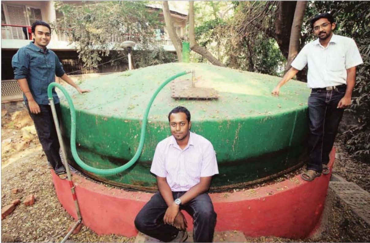
The biogas plant at the Tata Institute of Social Science was started with Rs 10 lakh approved by the institute.
